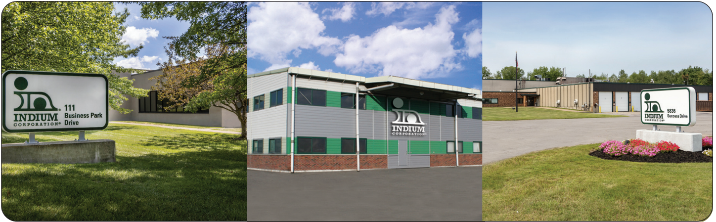
Above from left to right: Indium Corporation facilities in the Utica Business Park, South Korea, and Rome, NY.
