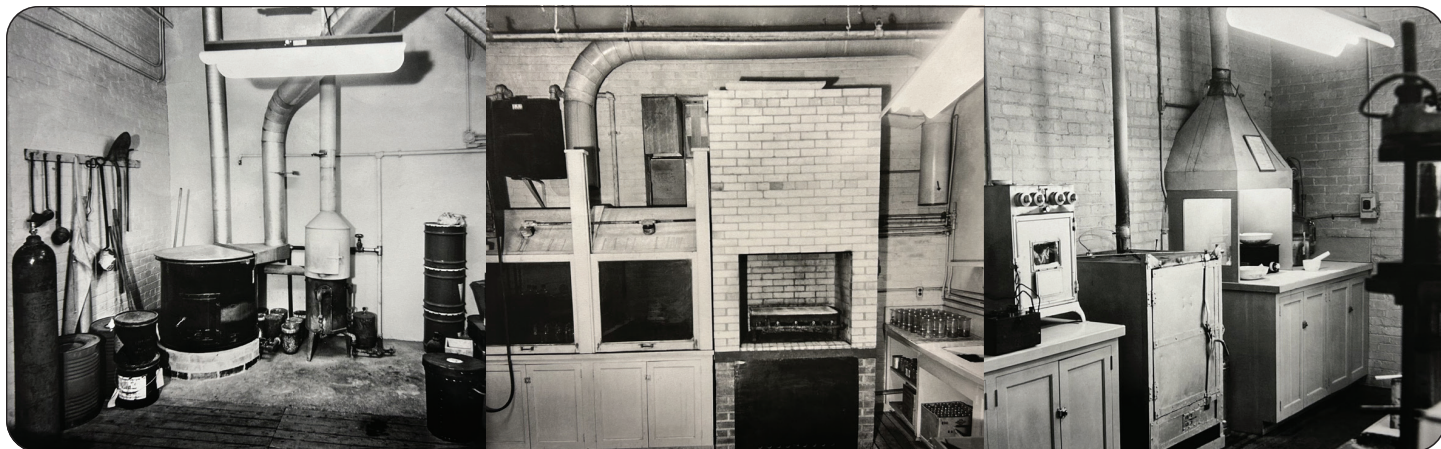
Historic photos of the interior of Indium Corporation's Lincoln Ave. facility.
